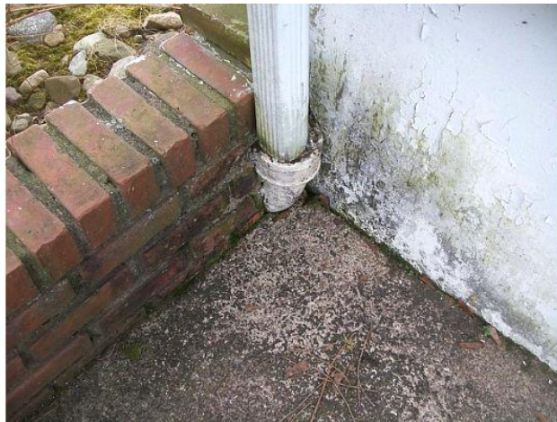
Old underground pipe
