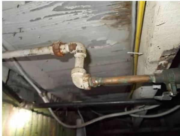
Old iron pipe attached to newer copper pipe
