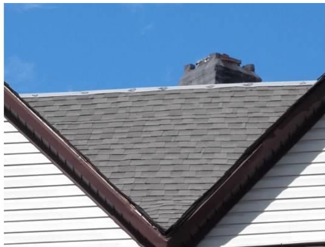
Patching along roof ridge
