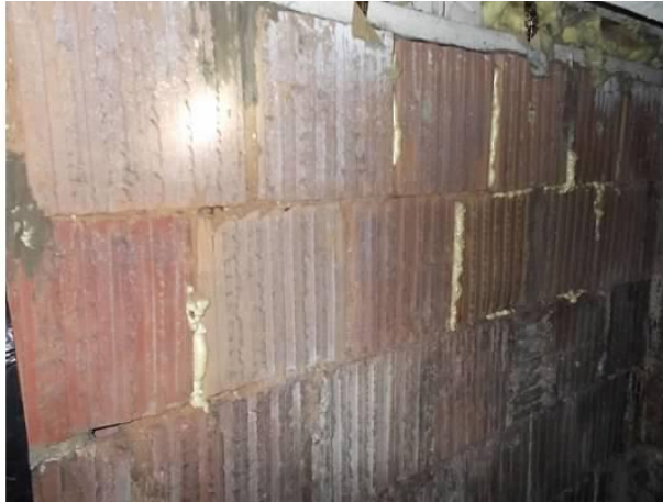
Spray foam between blocks
