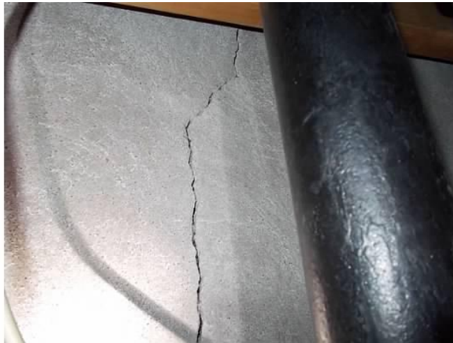
Vertical crack
